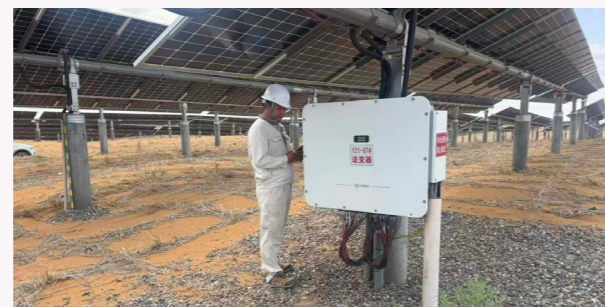
■ On-site Commissioning and Maintenance
