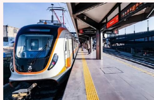
Guadalajara Light Rail Line 4 in Mexico
