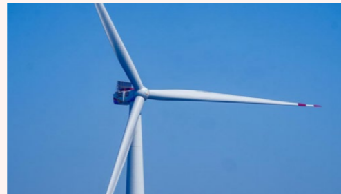
“Qihang” 20 MW Floating Offshore Wind Turbine
